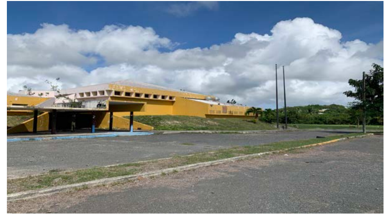
Top Existing Evelyn M. Williams Elementary School that will be demolished to make way for a new Arthur A. Richards PreK-8 building.
