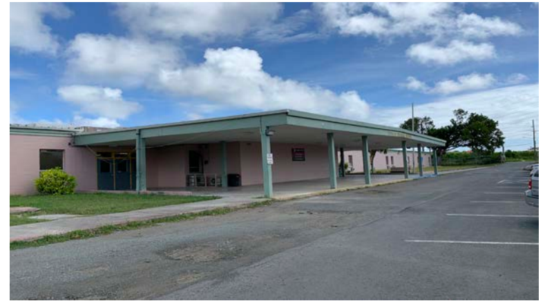
Top Existing Alfredo Andrews Elementary School that will be demolished to make way for a new Alfredo Andrews PreK-8.
