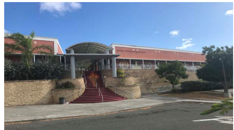
Bottom Existing Bertha C. Boschulte Middle School that will be renovated.
