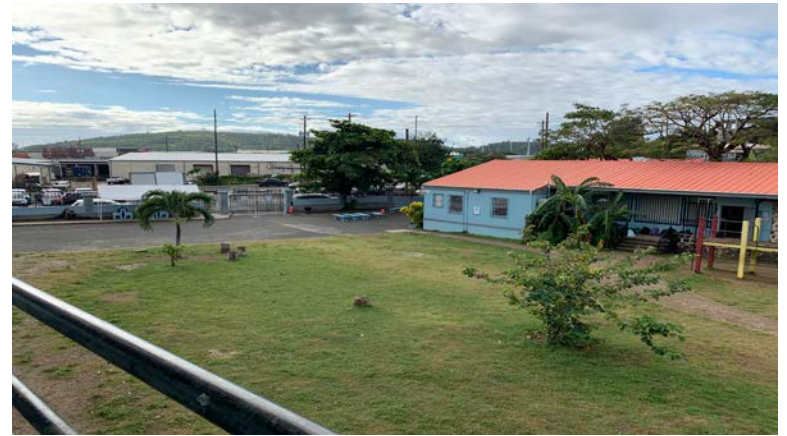
Top Existing Ulla F. Muller Elementary campus that will be demolished to make way for a new Ulla F. Muller PreK-8 building.
