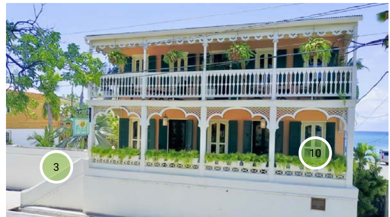
Bottom The Fred Boutique Hotel, Frederiksted, St. Croix
