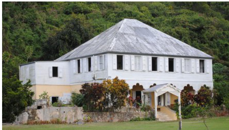
Lower Right Figure 19, 12 King Street, Frederiksted, St. Croix The Vernacular Architecture of Frederiksted, Robert S. Brown
