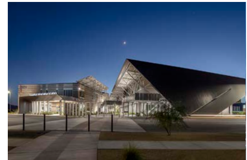
Canyon View High School Waddell, Arizona
